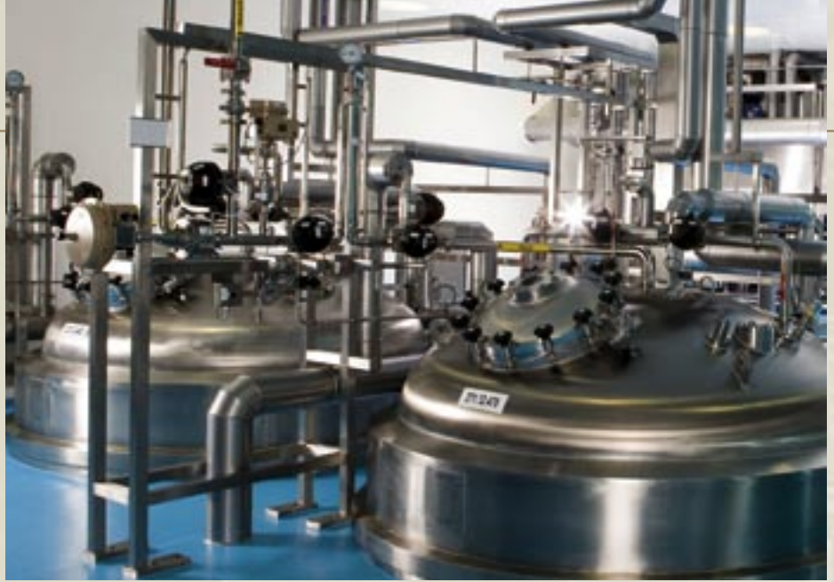
To ensure that chemical reactions run as required, complicate temperature profiles are often specified. The TROVIS 6495 is the right choice for the precise temperature control of reaction vessels.
