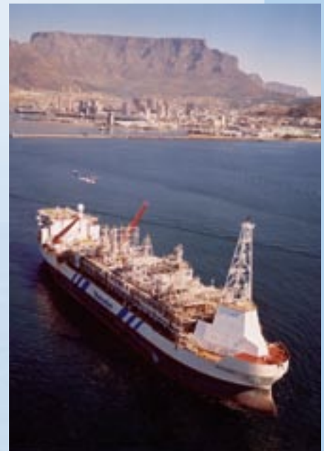
The FPSO Glas Dowr was fitted in Cape Town, South Africa and operates on the Sable field, 150 km south-west of Mossel Bay.
