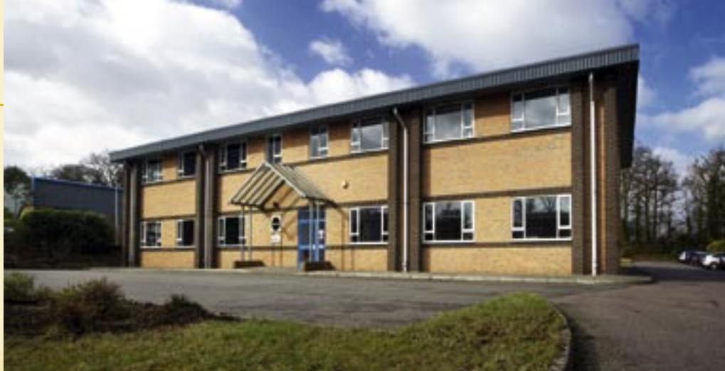
Headquarters of SAMSON Controls in Redhill near London.
