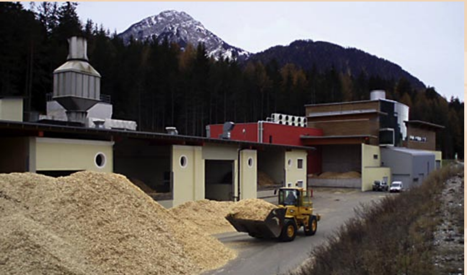
Hog fuel for the district heating plant is made from the wood waste produced by the local sawmills.
