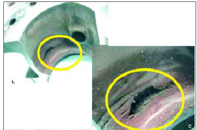
Fig. 14: First blowout and unpredicted plant shutdown
