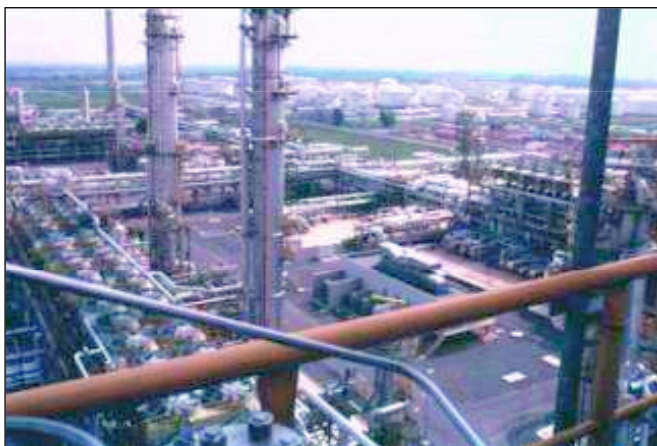
Fig. 13: TOTAL refinery in Spergau
