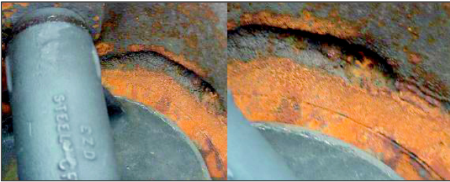
Fig. 15: Spare rotary valve under operation before replacement with 12" globe valve (just before the second blowout)
