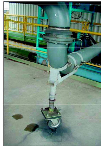
Fig. 26: Operating data show severe cavitation for standard type of rotary valve which increase noise to 96 dB(A) and cause severe vibration of the pipework
